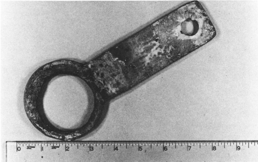
FIGURE 1-5 A slip-plate left in position for many months had corroded right through.
